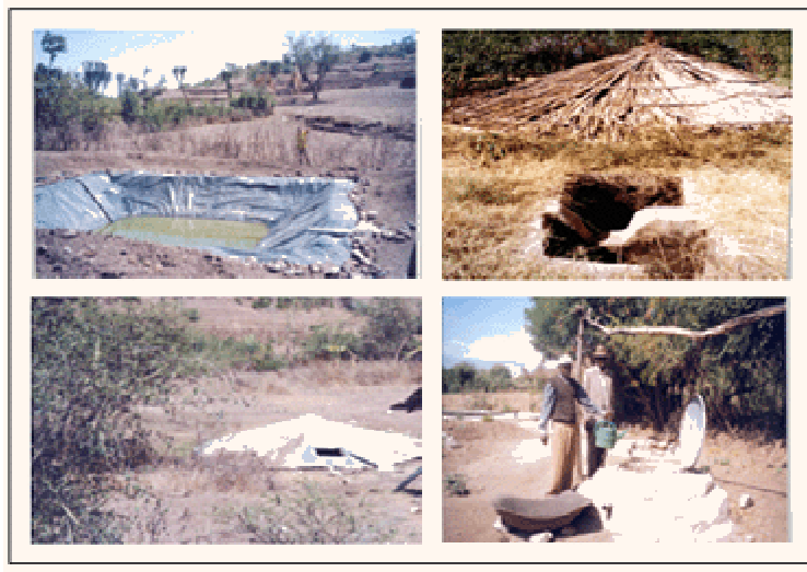
Figure 7: Types of pond covers in the study area. Clockwise from top left: the commonest type of pond; a cover made of thatching; a bottle-shaped pond covered perfectly with cap (expensive and rare); a covered made of corrugated iron.
